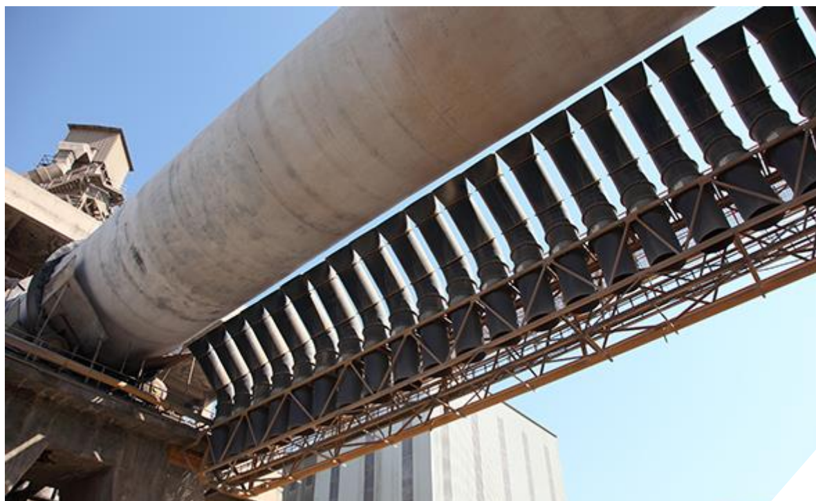
Mill Close up – Matola Plant – Mozambique
