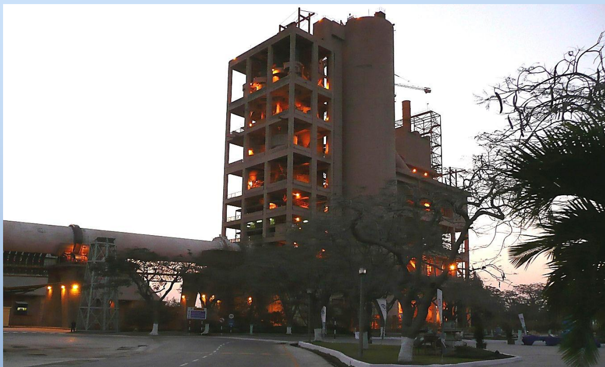
New Cement Grinding Mill – Matola Plant - Mozambique
